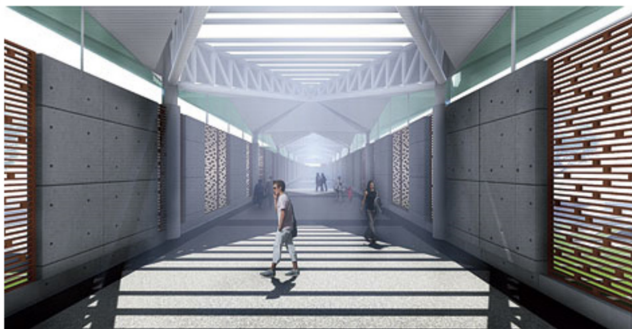
The entrance level will have perforated walls for ventilation. In the old design, there were no perforations. "This has been done to save energy," said architect Dey. The concourse level below will have air-conditioning
