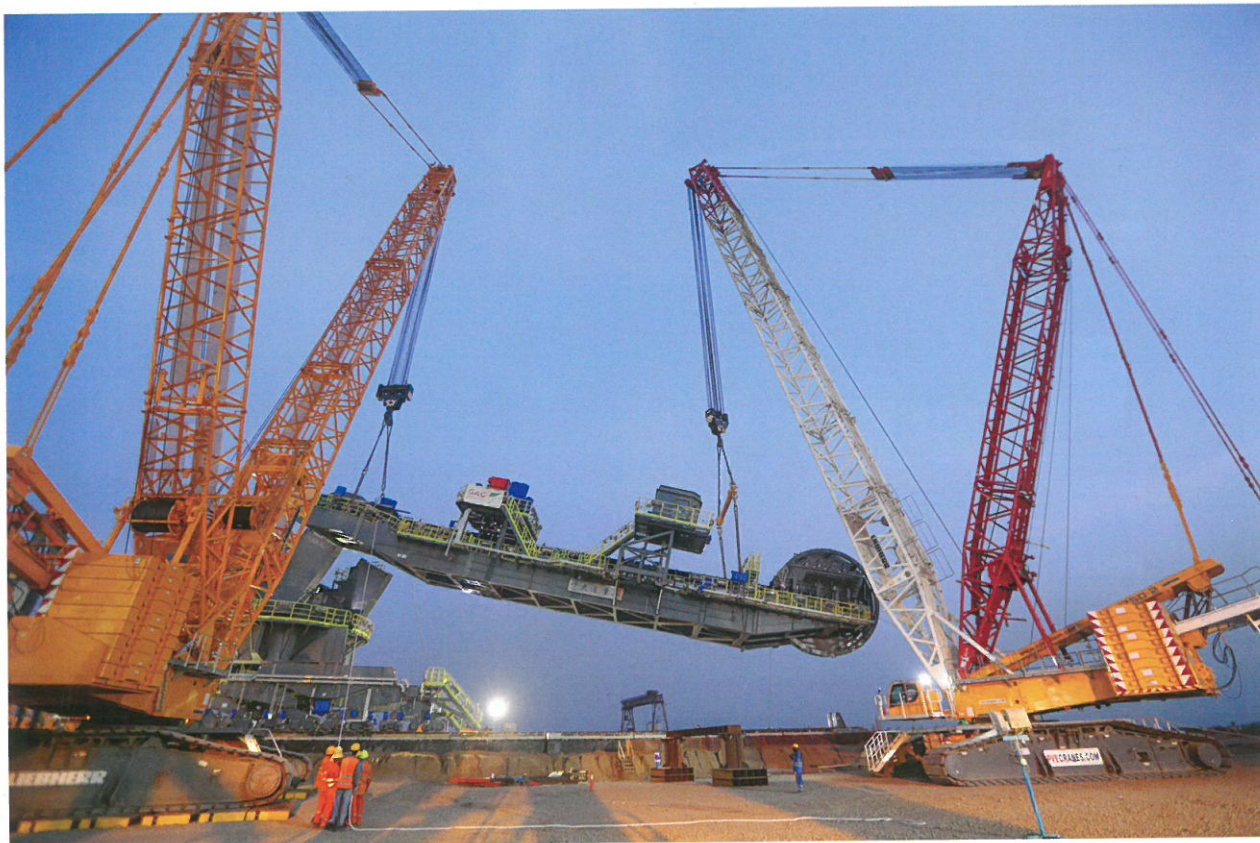
▲ Afcons' maiden project in Guinea where it set a record of carrying out the company's heaviest lifts while putting together the stacker reclaimer.
