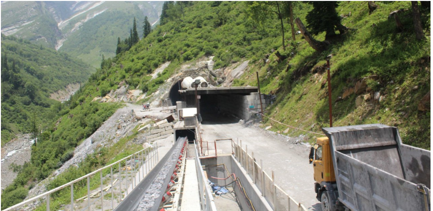
A view of the Rohtang Tunnel. Credit: DH File Photo
