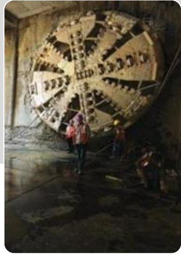
16 Tunnel Boring Machines (TBMs) +4 Pending Delivery
