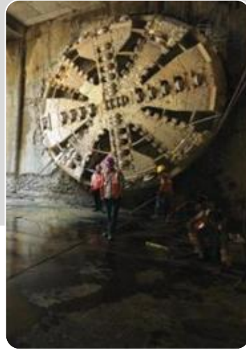
17 Tunnel Boring Machines (TBMs) +3 Pending Delivery
