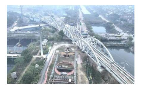
One of the challenging tasks in the package was the installation these six special bowstring steel spans on the corridor. These spans were erected amid heavy traffic congestion over road crossing and an irrigation canal in Kondli in East Delhi. The erection was carried out, in close coordination with NCRTC, with meticulous planning and precision.
