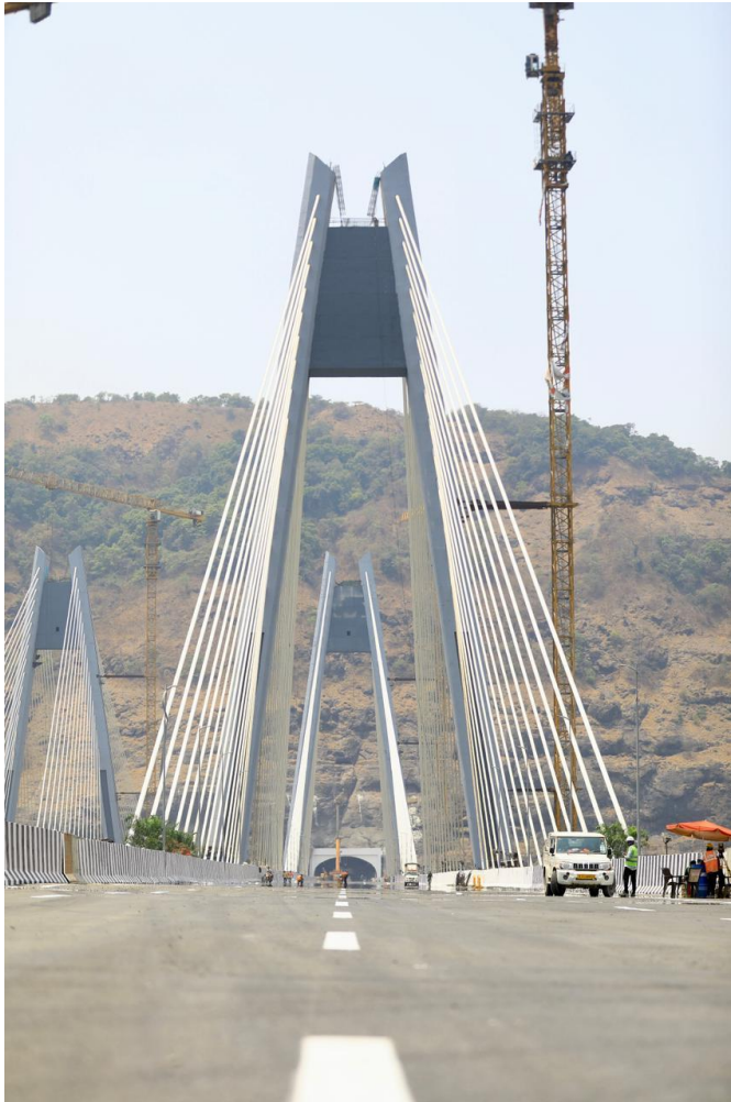
Caption – panoramic view of India's tallest road cable stayed bridge of Missing Link
