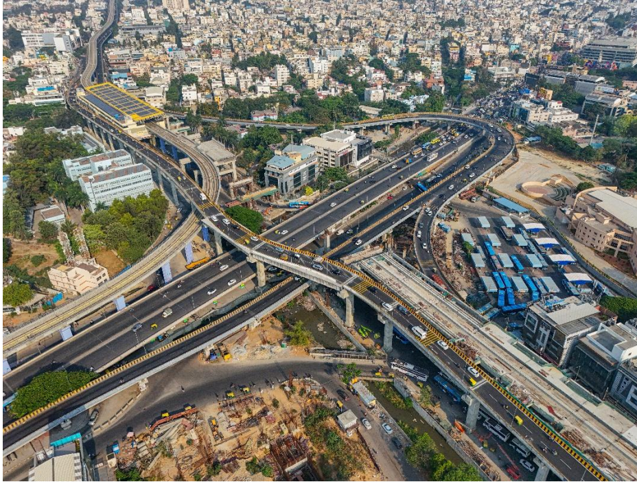
Photo caption – D & E flyovers of Central Silk Board Double-Decker flyovers in Bengaluru opened for public today
