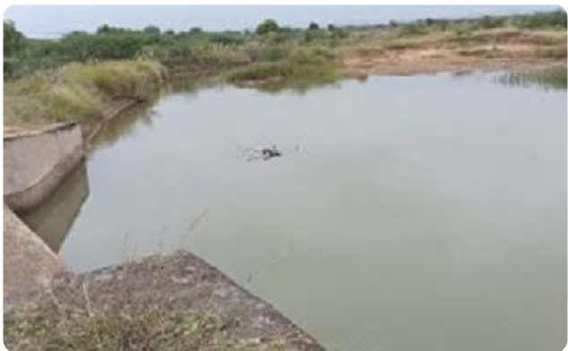
Facilitated construction of eight check dams across Rajasthan, building a total water harvesting and groundwater recharge capacity of 102 crore litres.
