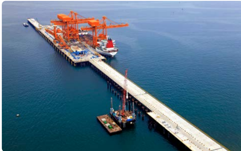
Bulk Jetty, Port of Sohar, Oman
